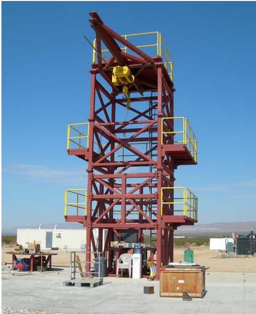
Vertical test stand completed
