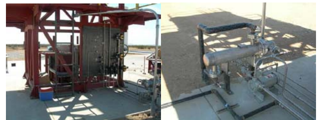
Vertical test stand electrical & plumbing installed
