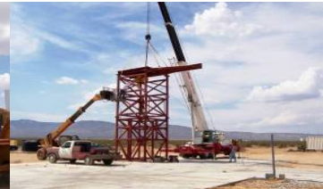
Last tier in place
